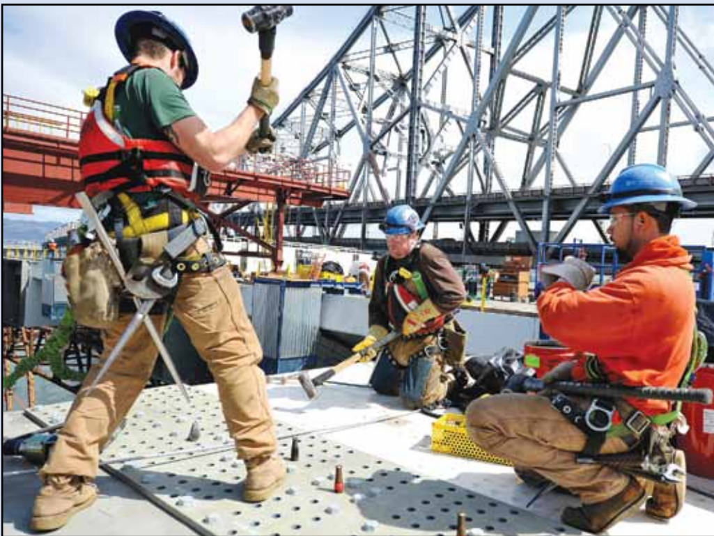
Three Ironworkers, including Jake Mesche and Darryl Webb, work together to drive pins into a crossbeam, 2010.
